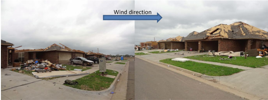
Fig. 14.5 Failure of roofs and garage doors on different sides of Kyle Dr. (camera pointed to the north)
